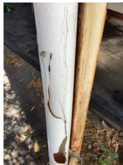
Broken downpipe.
