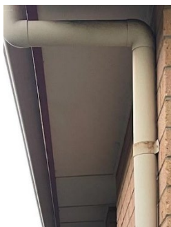
Clear and functioning downpipe elbow.
