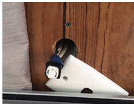
Exposed wiring
